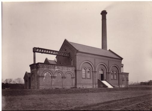
The two engines and boilers, for raising steam, were housed in a building erected by Thomas Lowe and Sons. Although not especially architecturally interesting, the station with its tall chimney stack remained a landmark for railway passengers travelling between Lichfield and Burton on Trent until Dr Beeching axed the service in the 1960s.
