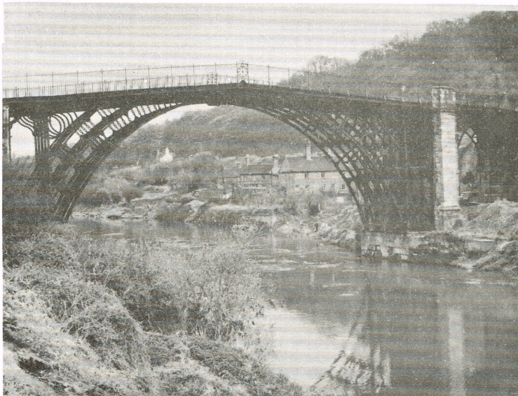
The first cast iron bridge in the world built to span the River Severn at Ironbridge, Salop
