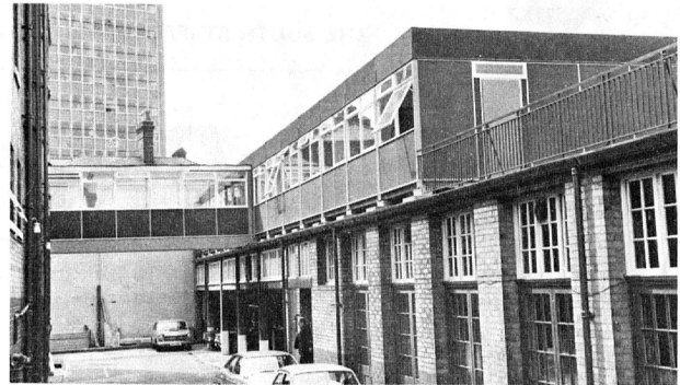
New C.E.D. building on canteen roof with link bridge to main offices.
