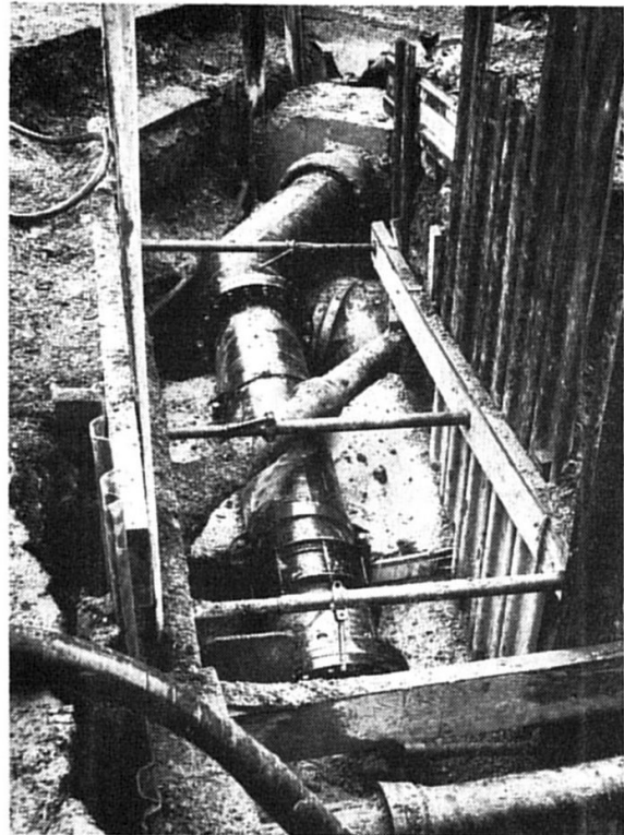
The last link from Severn to Blithe . . . a 450 mm bypass
