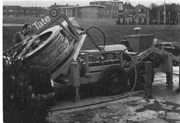
Scraping and re-lining (see page 6).
