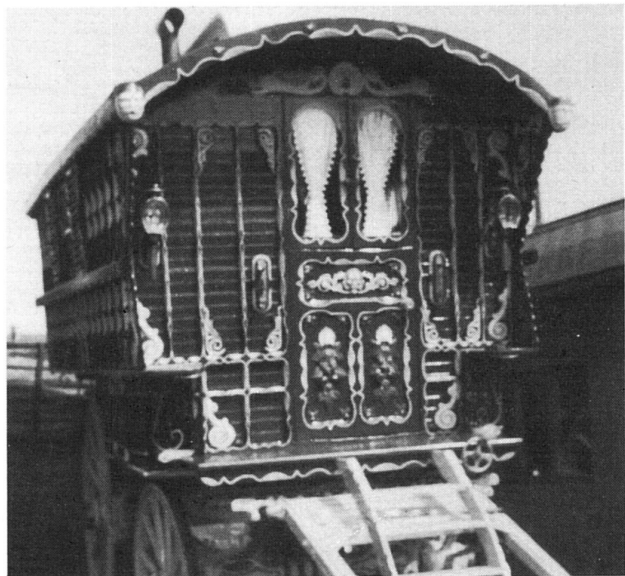
The renovation complete
