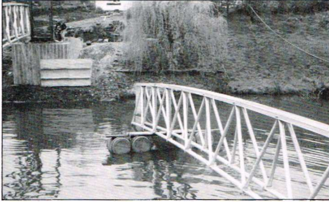
Above... One member being floated into position.
