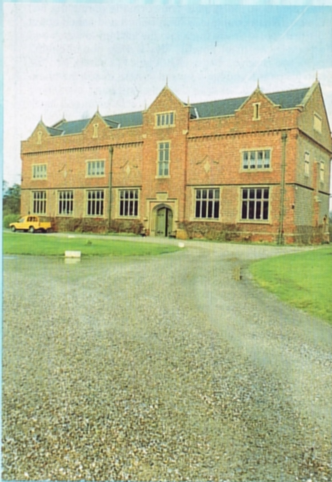
Brindley Bank Pumping Station Victorian Architecture at its best
