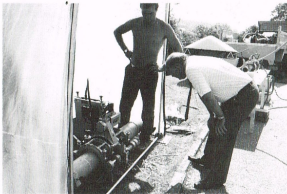
Jim - prominent as ever - on site at Little Hay.
