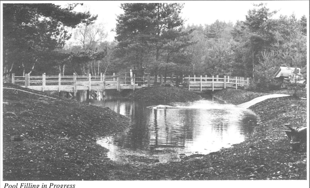
Pool Filling in Progress
