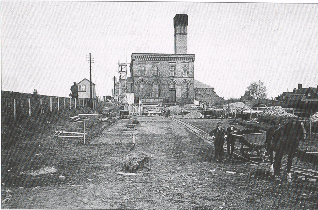
Work commencing on the treatment works at Sandfields in 1923
