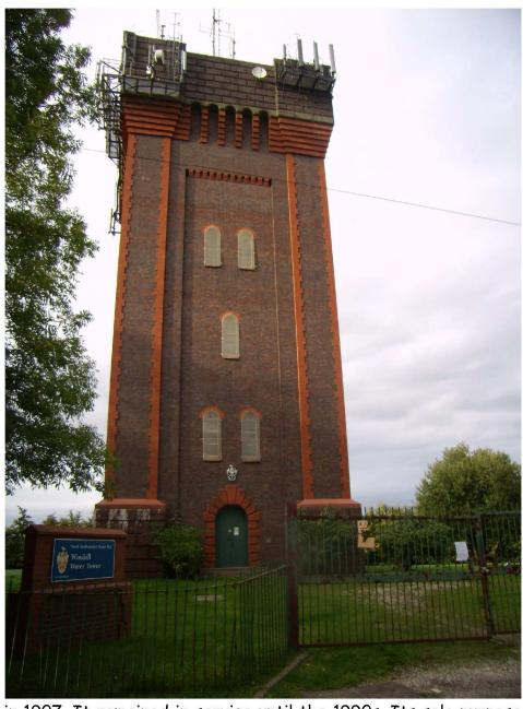
Winshill Tower was the first tower to be built by the Company and was completed in 1907. It remained in service until the 1990s. Its sole purpose today is for the accommodation of third party radio communications equipment and associated aerials which festoon the roof of the tower.
